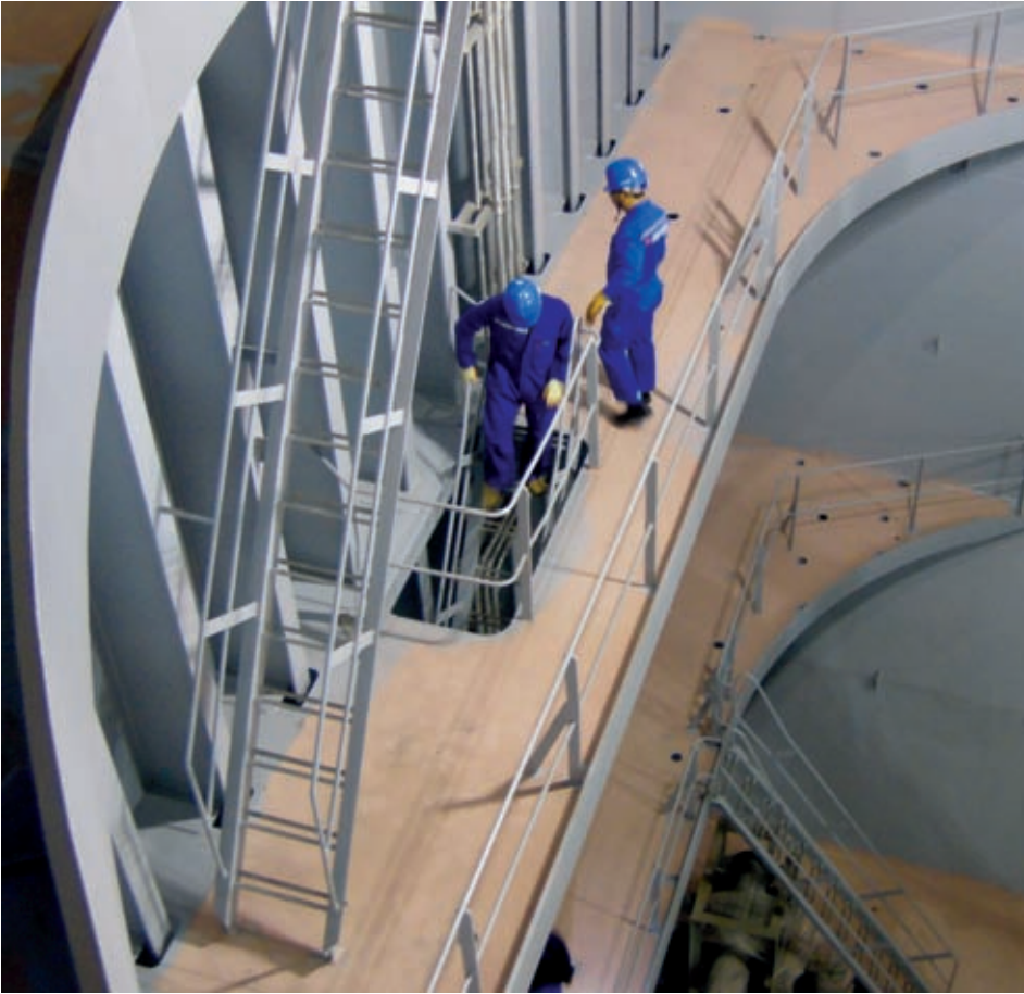
IP's new tank coating could last for up to 15 years.
