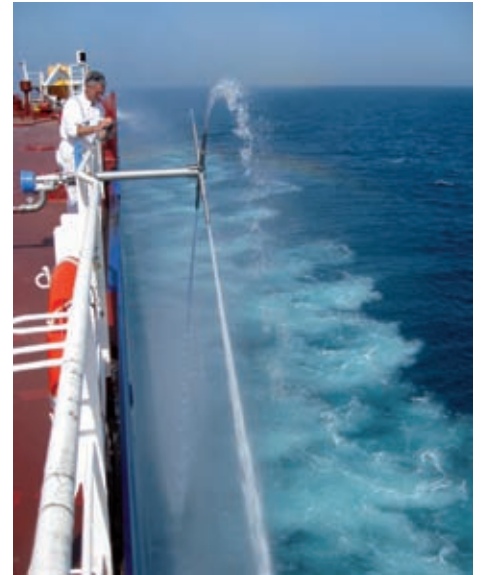
There should be a strong water beam emitted.
